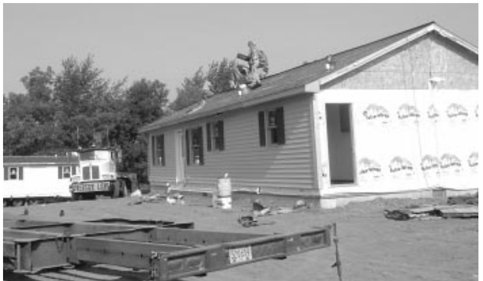
Workmen put some finishing touches on House G
